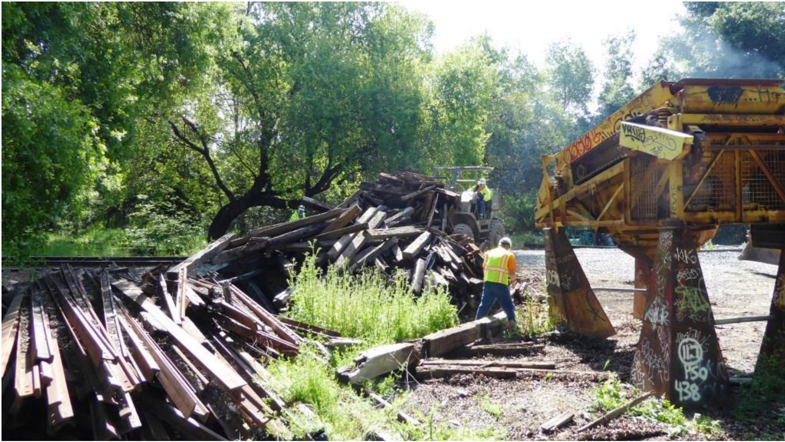
Mike F. digs into the side of Mount Tie Helens with the forks of GM2 as John attaches a chain to a bridge timber from the turntable
