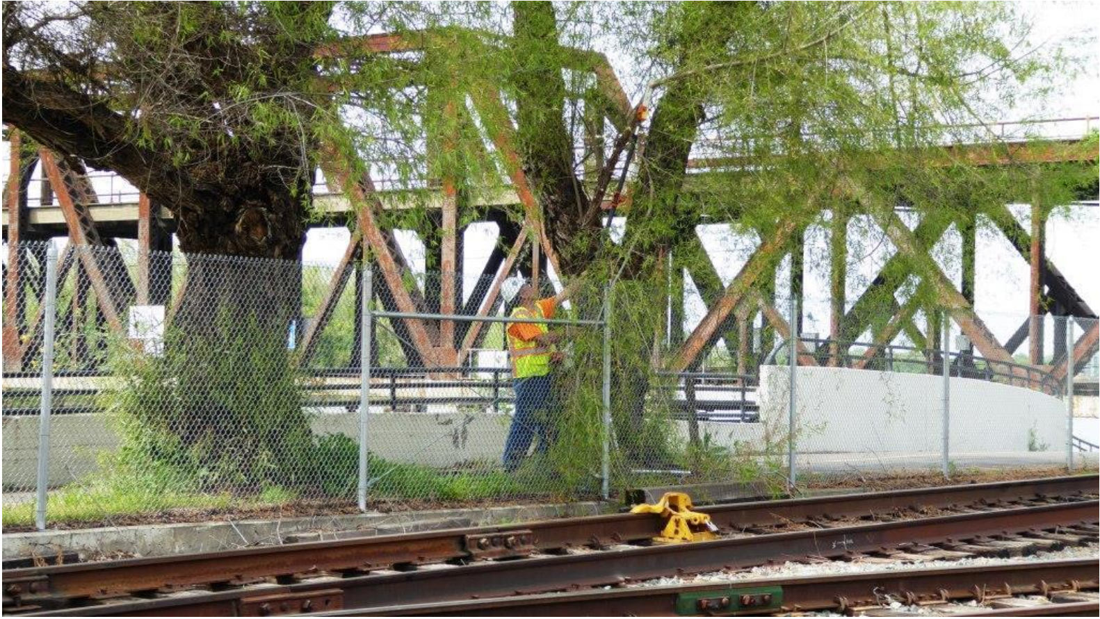
John uses the gas-powered chainsaw-on-a-stick to remove offending branches over the 150 Track
