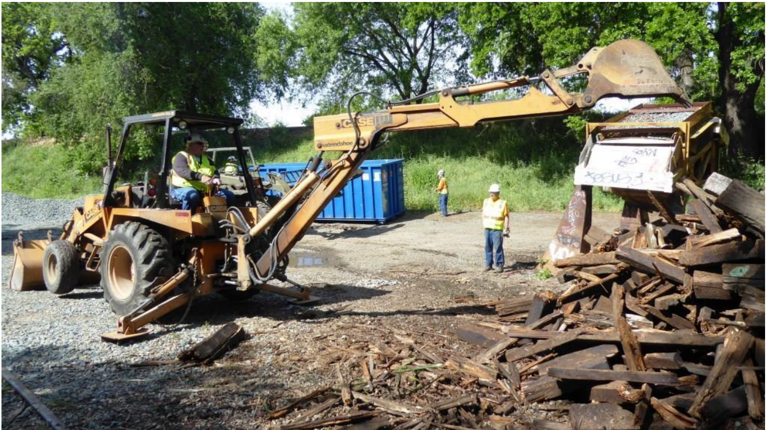
Harry used the extend-a-hoe on the back-hoe to dig into the tie pile and pull some of the big ones off the top
