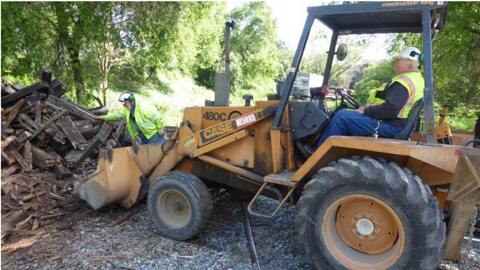
Harry brings in the back-hoe as Frank loads tie pieces into the bucket
