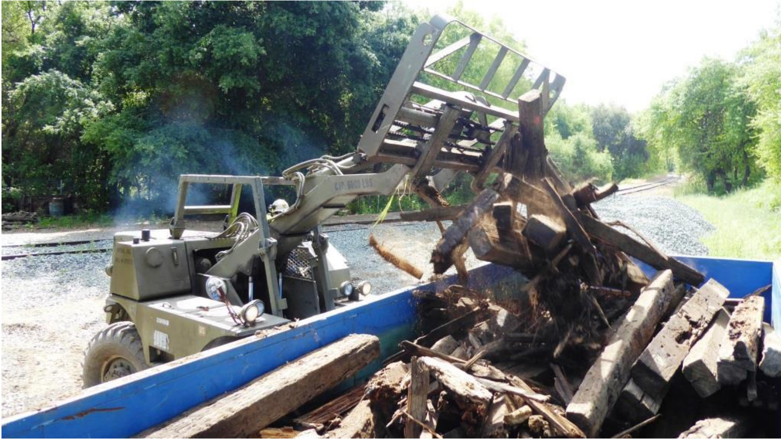
GM2 drops a load of dead-ties into the dumpster
