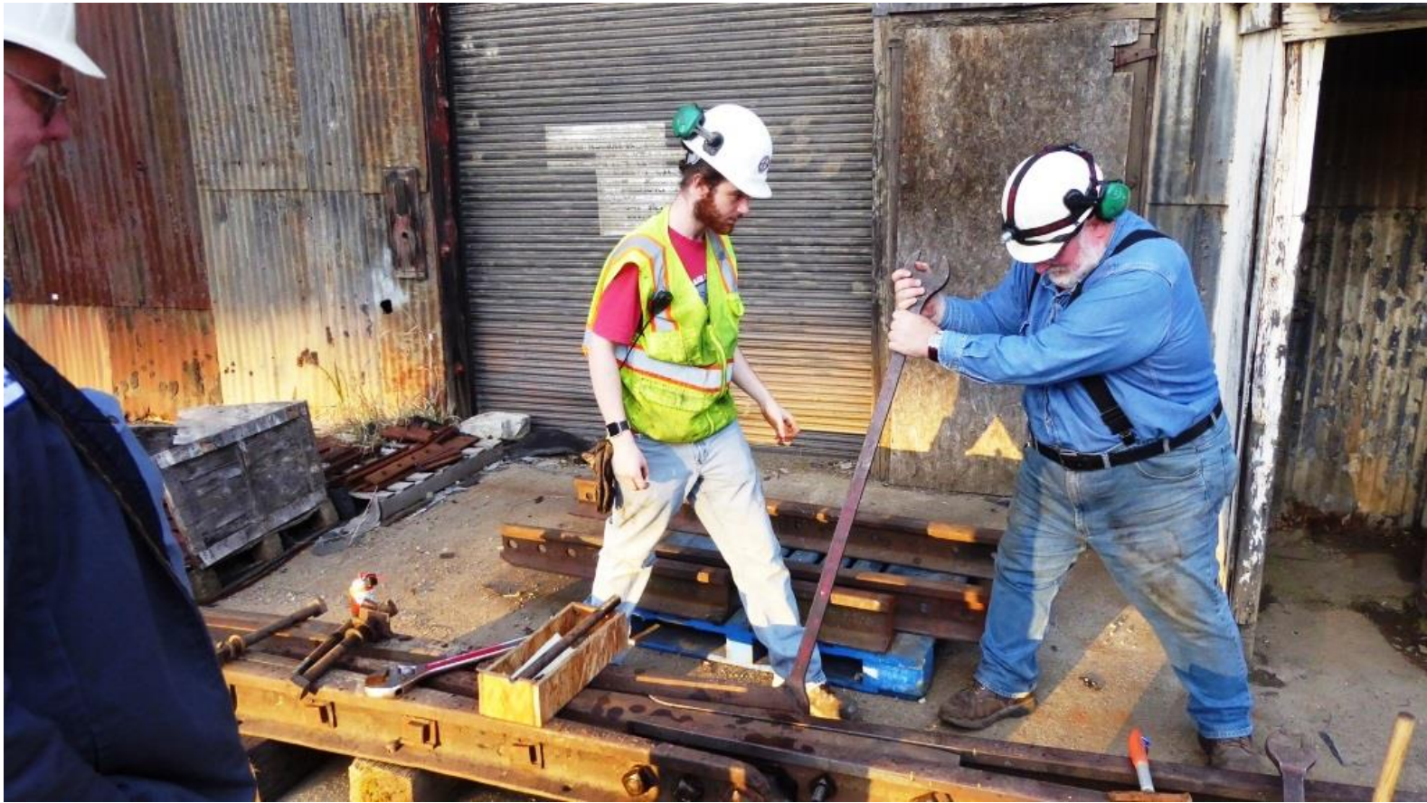
First Matt and Frank try to close the gaps between the frog and wing-rails by tightening bolts...
