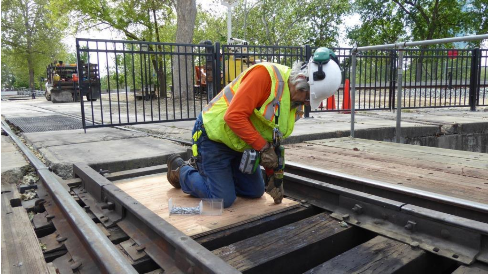
Ed secures the new panel to the ties of the turntable
