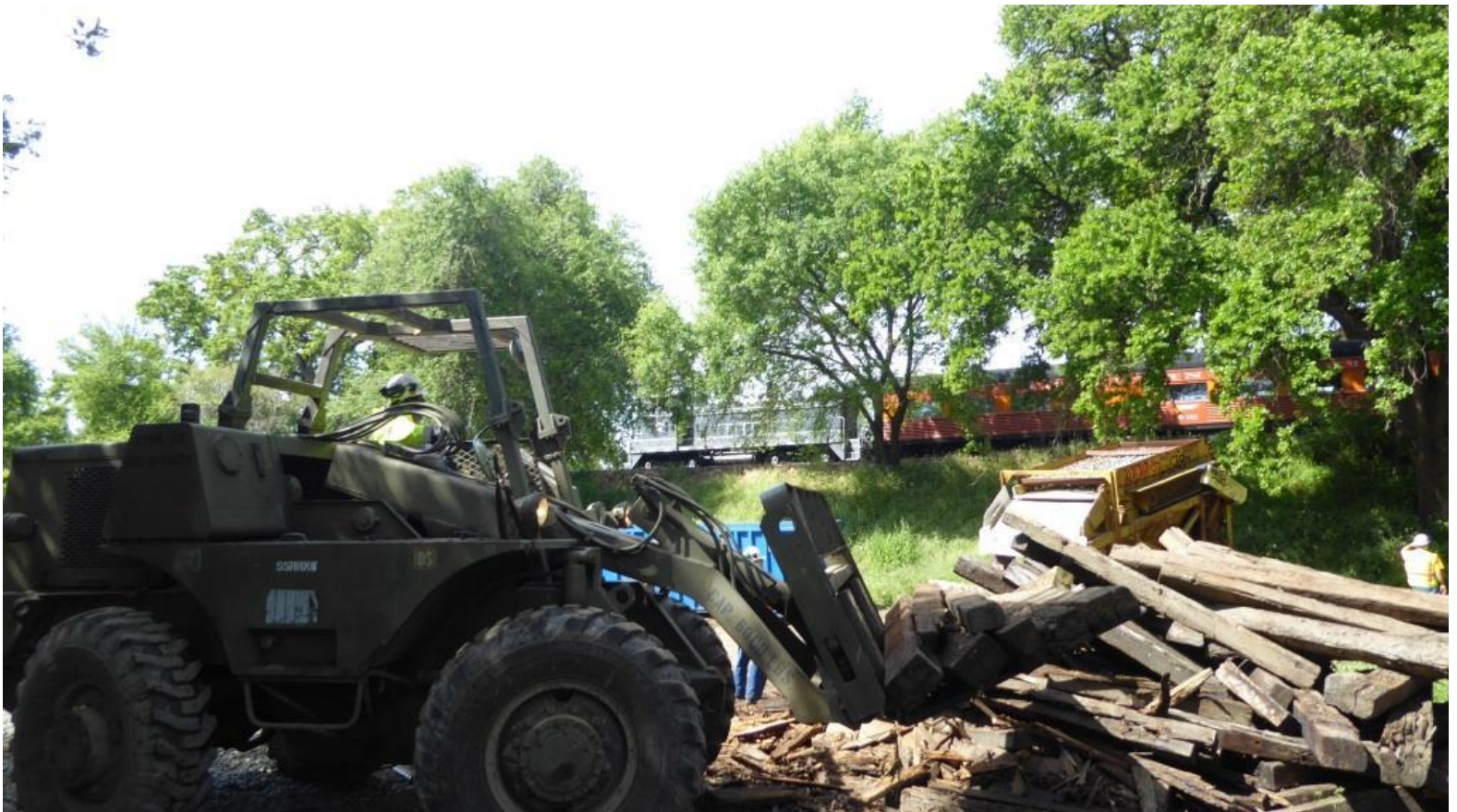
First train of the day rolls past our work-site
